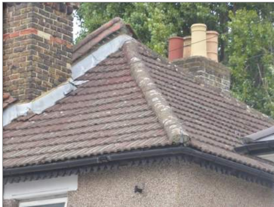
Photo - 4 Main roof covering- fair order
